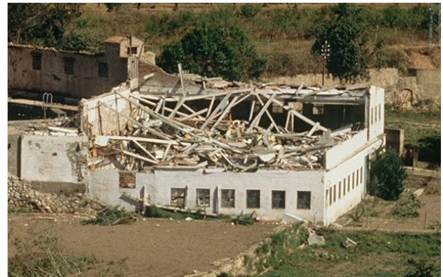
Fig. 2. Example of the impacts produced by a tornado: collapsed farm caused by a tornado in Espluga de Francolí (Spain), on August 31, 1994 (photo © Miquel Gayà).
